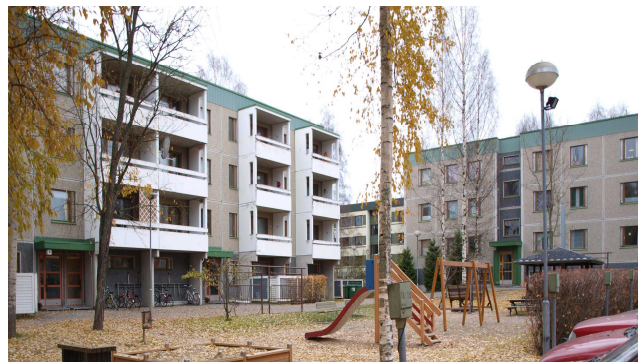
Figures 1 and 2: A significant number of suburbs were constructed in Finland in the 1960s and 1970s in which multi-storey apartment buildings constructed of prefabricated concrete elements are the dominant building type.
