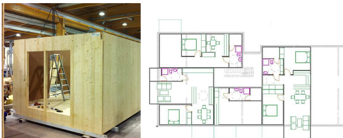
Figure 7 and 8: Left, fabrication of CLT module elements. Right, a plan for an additional storey made of prefabricated module elements.
