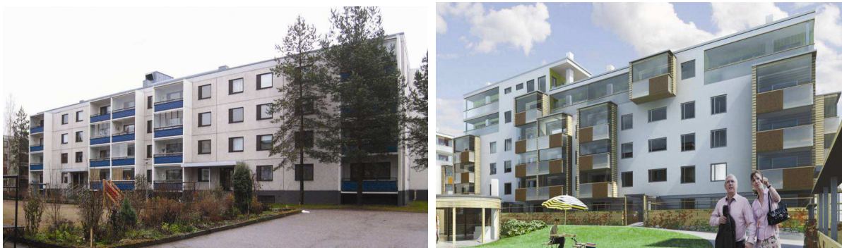
Figure 3 and 4: In Riihimäki the possibility of raising the four-storey buildings to cover the renovation cost and to improve the milieu has been examined. Present situation at the left. (Tomi Tulamo's master thesis, Aalto University 2010)
