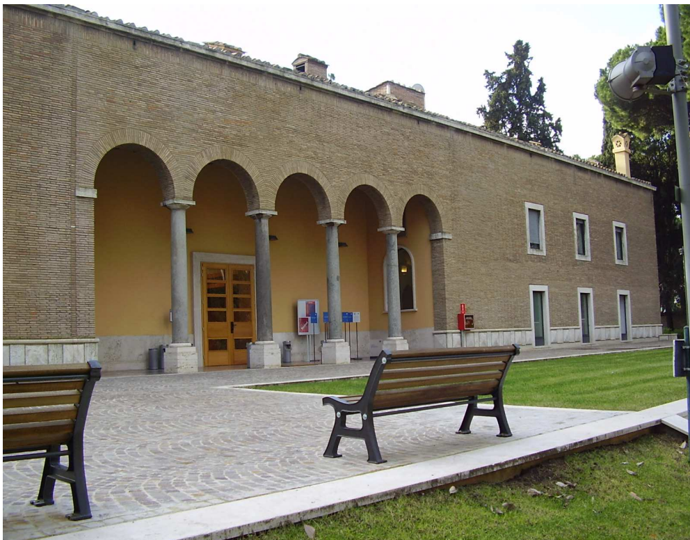
Figure 2: Main entrance to the concert hall ('A' building) (Biocca, 2006)
