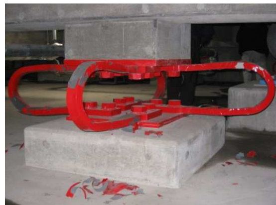
(b) U-shape steel damper
