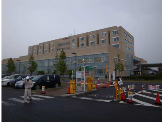
(a) Overview of the building
