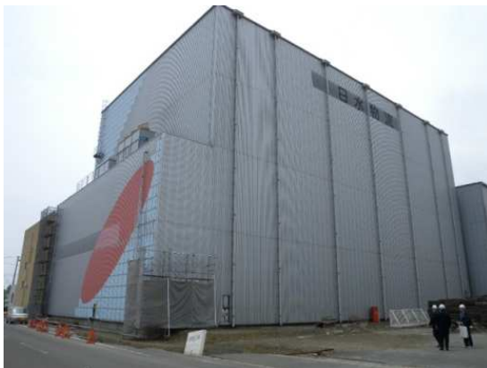
(a) Overview of the building
