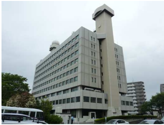
(a) Overview of the building
