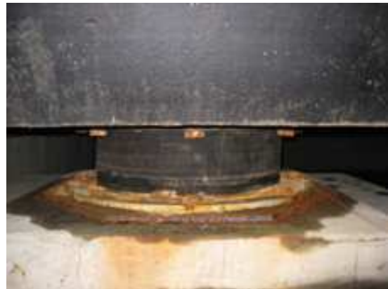
(b) Damage to the cover panel
