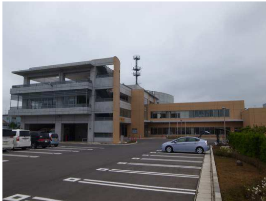
(a) Overview of the building
