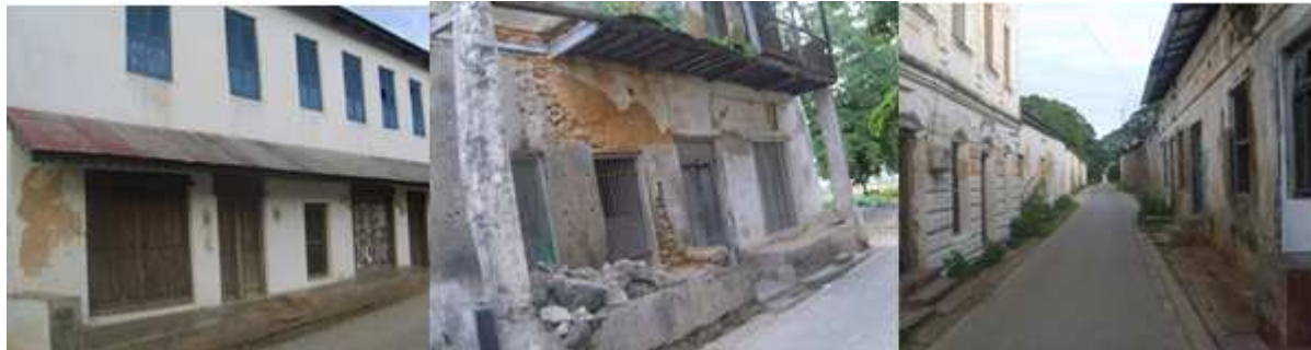
a) Roof overhang, elevated plinth and lime-based coating
