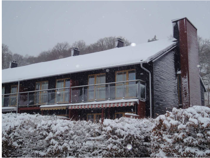
Figure 1. Clear formulation of requirements provides the basis for successfully achieving an airtight building. The Lindås houses are an example of such a project, in which requirements were formulated and monitored.
