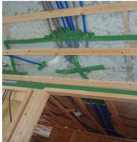
Figure 2. Penetrations through the sealing membrane can be avoided if the membrane is applied in such a way as to leave a gap for installation of the building's services systems.
