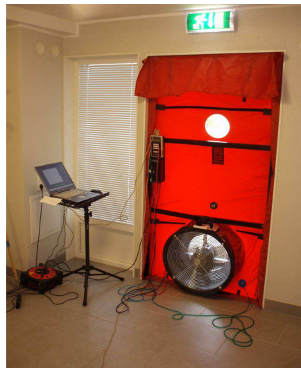
Figure 3. An airtightness test (Blower-Door), looking for air leaks, provides indication of whether the requirements have been fulfilled.
