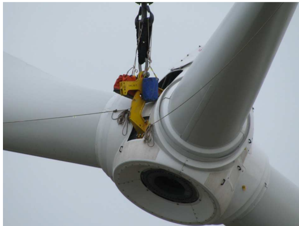
Figure 3. Customized Crane Attachment for Hoisting Main Hub into Place
