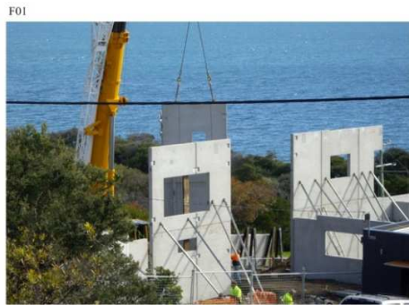
Description: Precast concrete panel system for housing Source: By courtesy of Mark Vines of RMIT University
