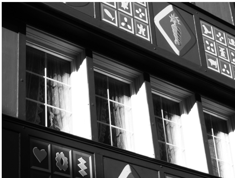
Figure 4. A residential building from 17 th in Appenzell, Switzerland after a “Sanierung” with a new coat of paint and new windows (NB. Plastic bars, without function, behind a single glass pane)
