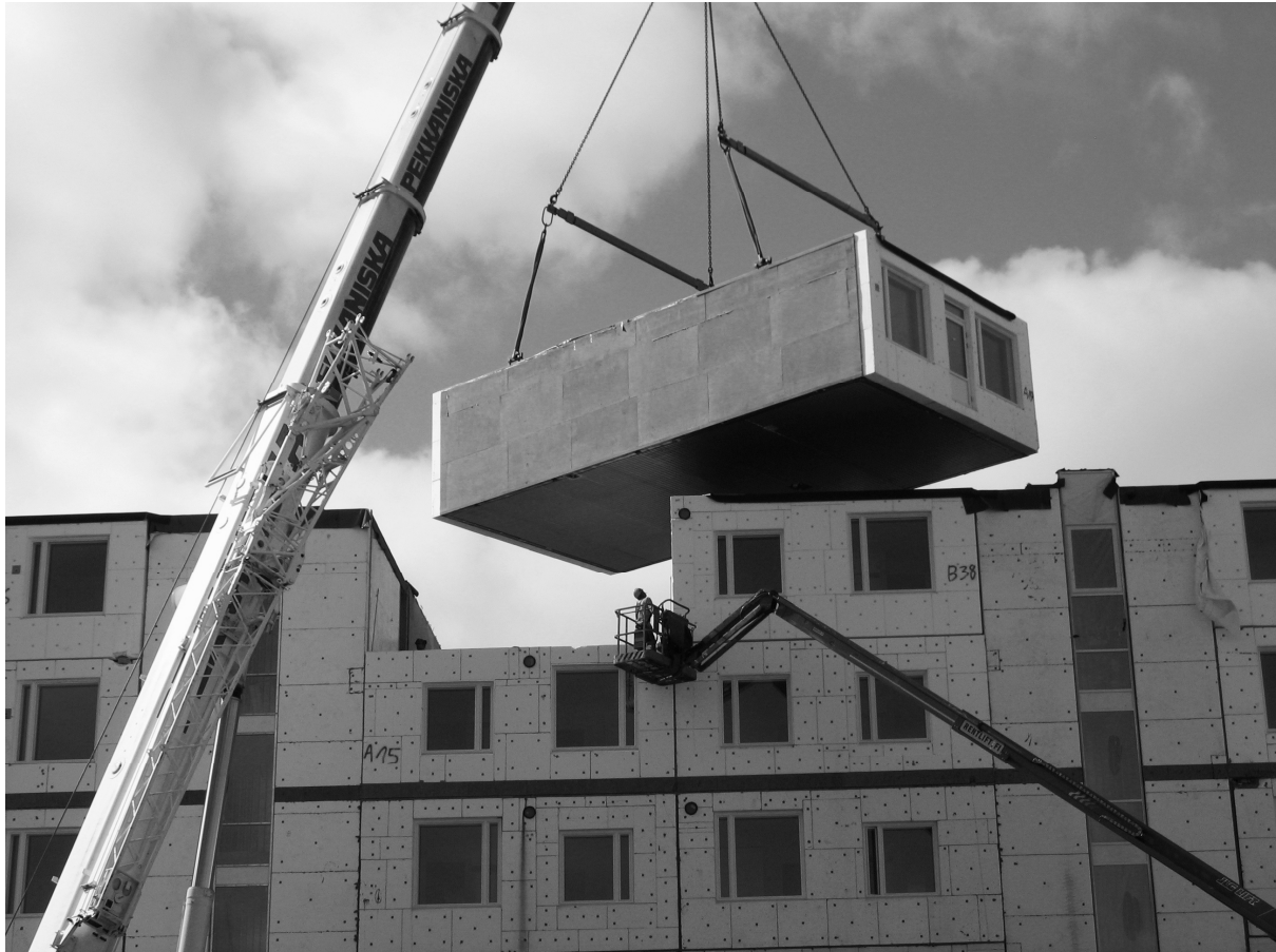
Figure 2. Installation of cellular modules for the case project B.
