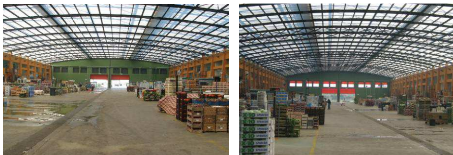
Picture 1: Central gallery overlooking the West (left) and East (right)
