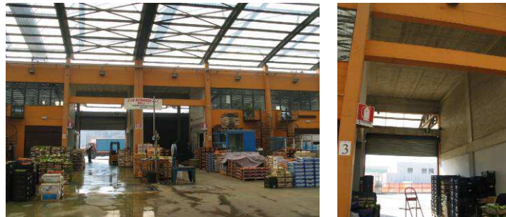
Picture 2: Box at the sides of the tunnel (left) e inside the box (on the right)
