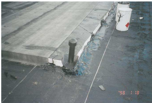
Picture 13: The lying of second layer of bituminous membrane, with mineral surfacing, was done as soon as slopes was wholly accomplished
