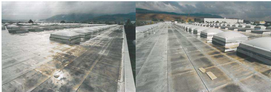
Pictures 4 and 5: After a rainfall, the covering presented itself as one immense quagmire
