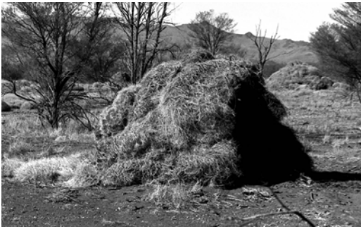
Figure 3. Spinifex grass was by far the most widespread resource for the cladding wet weather domes in the Western Desert. This example at the Tomkinson Range near the Western Australian border. (Photo by Howard Hughes, Australian Museum.)
