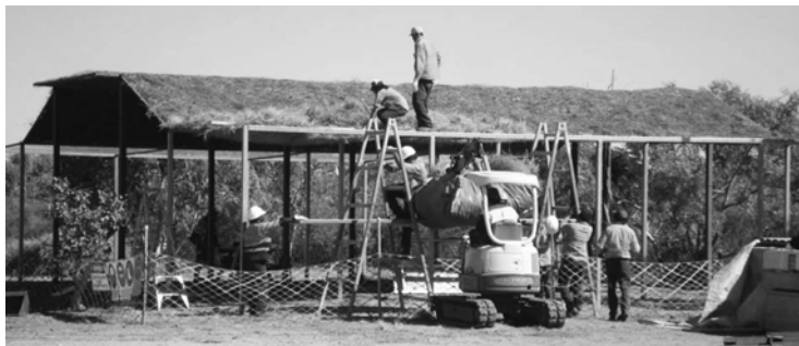
Figure 5. Modern remote spinifex bough shed construction at the Dugalunji Camp, Camooweal, North-west Queensland. (Photo by Tim O'Rourke.)
