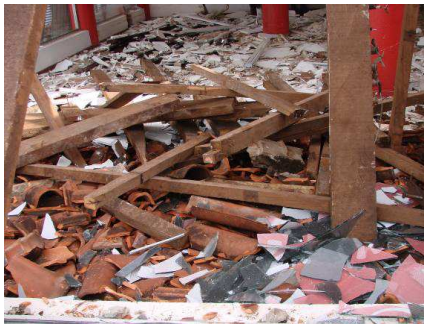
Figure 5 and 6: Mixed materials during demolition (Mattaraia 2012)
