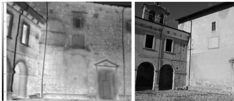
Figure 7. Santa Maria di Valleverde church in Barisciano, thermograph and photo
