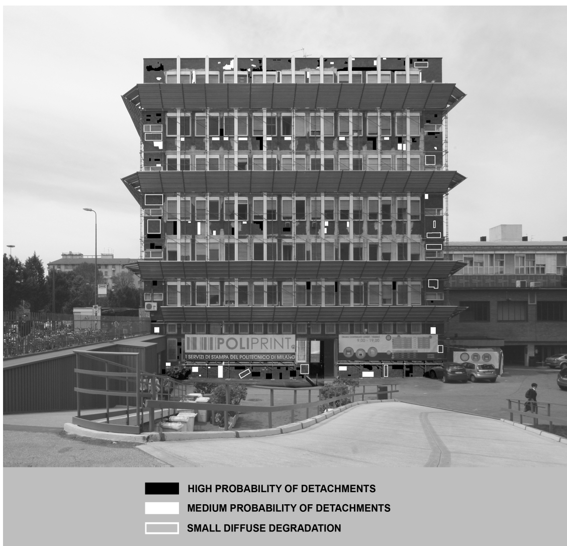
Figure 8: Example of application: Building 12 East façade, possible detachments of cladding tiles
