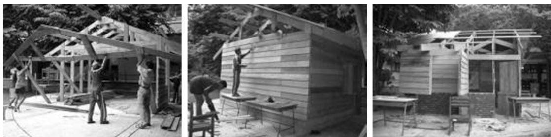
Figure 3: Construction Process of RIA (Silas and Setyawan, 2010)
