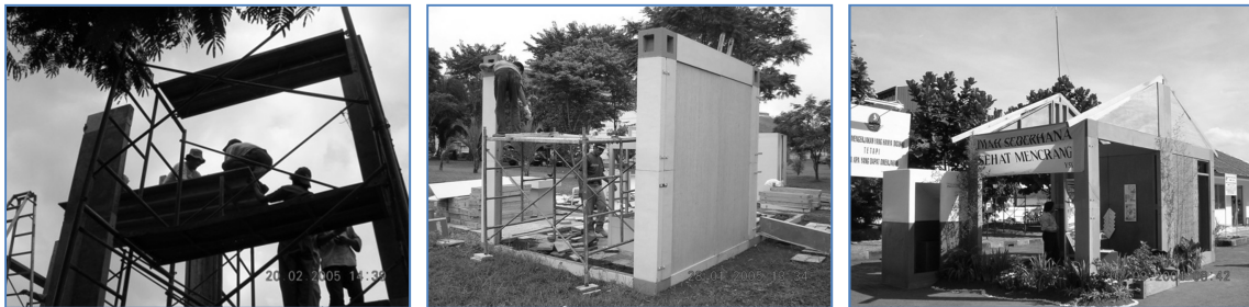
Figure 4: The construction process of RISHA house (Menpera, 2011)
