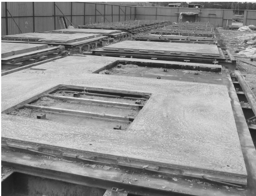
Figure 1: Precast wall panels at the casting yard
