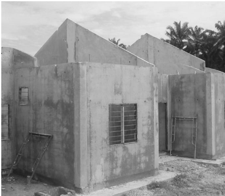
Figure 4: Completed precast wall panel with in-situ columns
